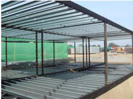
Welded module prior to fit-out
