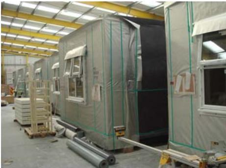
Modules with external joinery, sheathing and breather membrane fitted.
