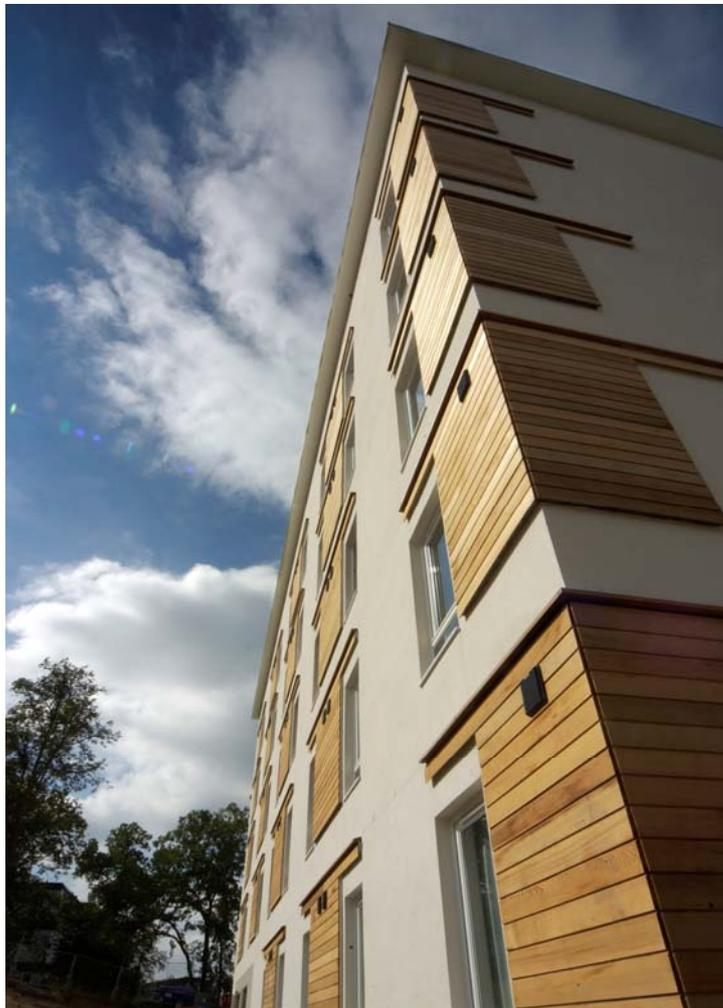
Volumetric construction reduced the waste generated in building multi-occupancy buildings to 5.5 m<sup>3</sup> per 100m<sup>2</sup> of construction: a reduction of 48% compared to traditional construction.
