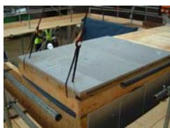
Floors can also be assembled at the factories into cassettes. Floor cassettes comprise a series of timber joists (solid or engineered timber). The platform is completed with weather protected chipboard fixed to the top of the joists.
