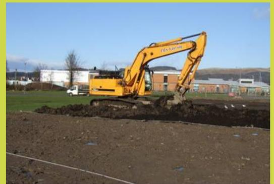
Figure 9: Compost being incorporated into a trial plot, Raploch
