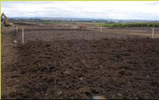
Figure 6: Trial block at the Ravenscraig site, shortly after the topsoil had been laid.
