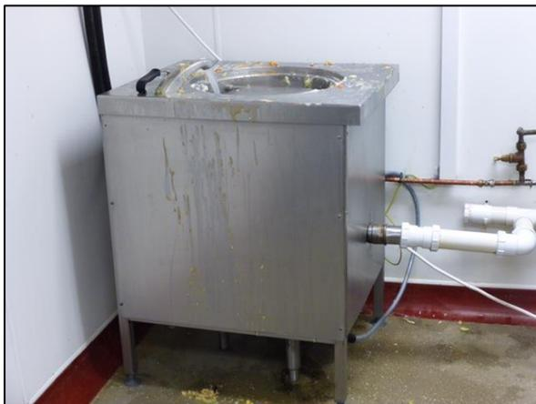
Figure 3: Macerator unit, used to dispose of food waste to sewer
