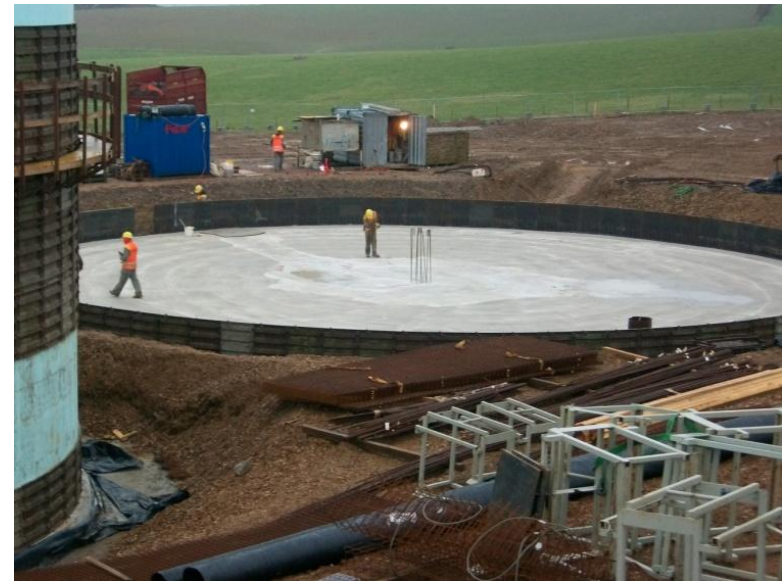
Langage farm under construction
