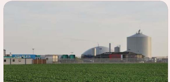
**AD facilities can provide heat and power as well as replacing inorganic fertilisers. For example, this Staples facility will produce 11 million kilowatt hours of electricity every year from 40,000 tonnes of vegetable waste**
