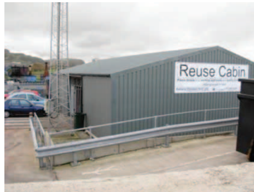
Reuse cabin at Seafield Community Recycling Centre, Edinburgh City Council
